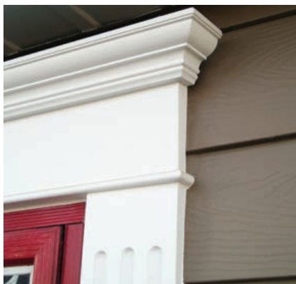
Cornice showing return
